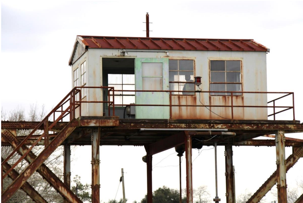
Condition Photo 19: Operator's house centered on top of the main truss span.
