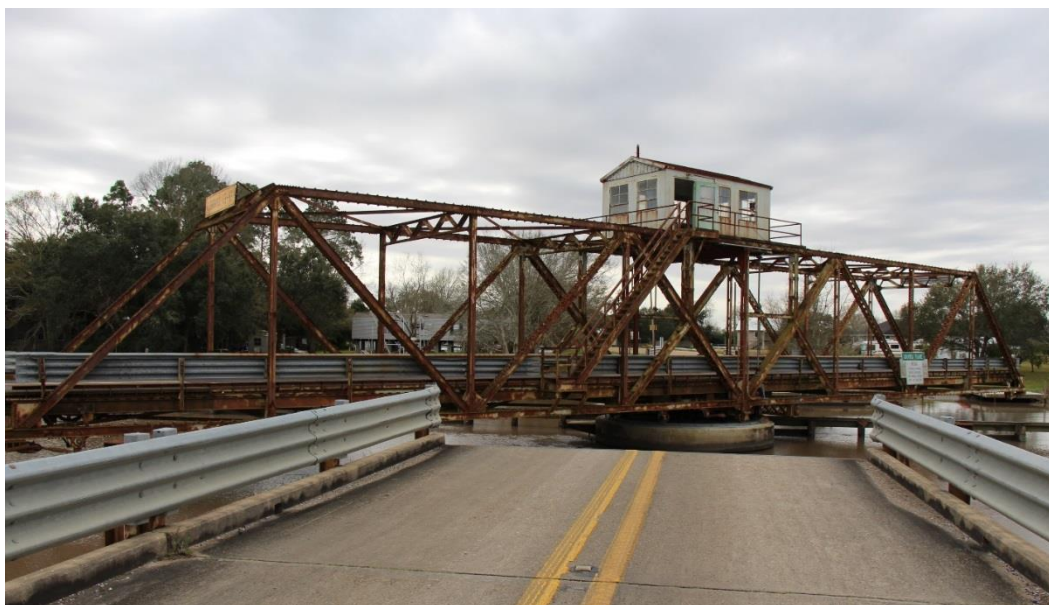
Character-defining Feature Photo 1: Design and construction of a through truss swing span. The main swing span (shown in partially open position) features a Warren through truss.
