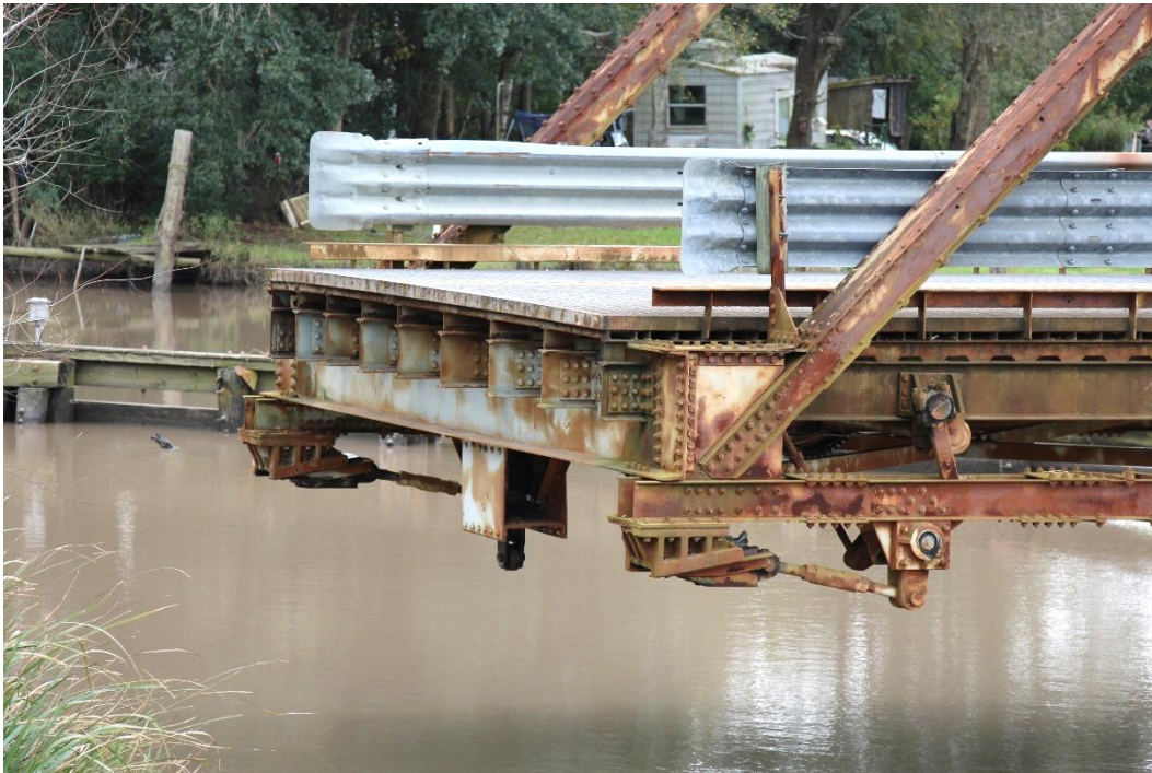
Historic Fabric Photo 1: Truss floor system.
