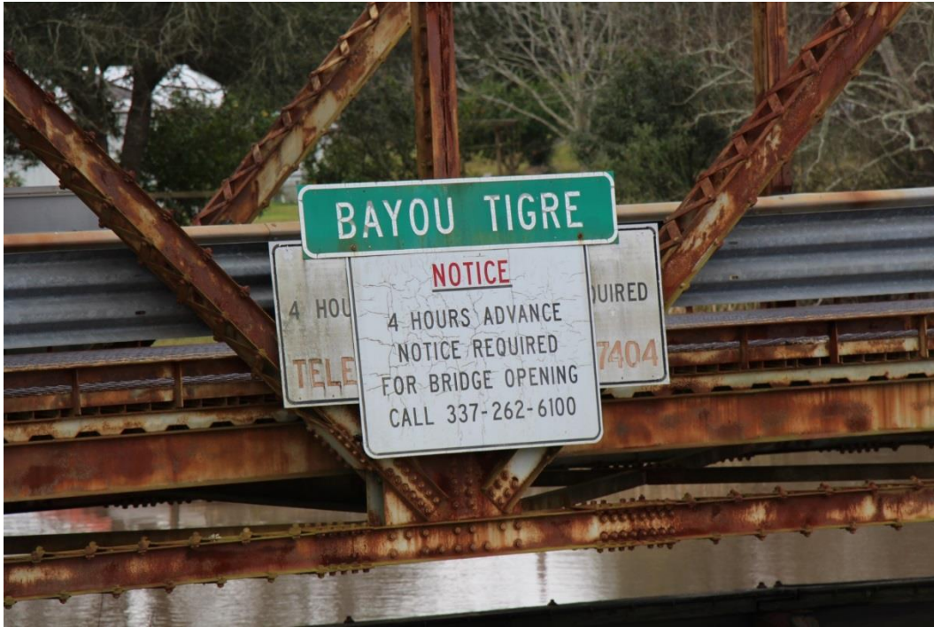
Condition Photo 12: Signage attached to a vertical member of the truss.
