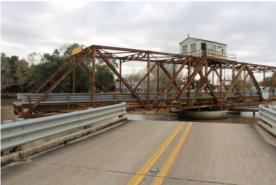
Condition Photo 7: Opening of the swing truss span.
