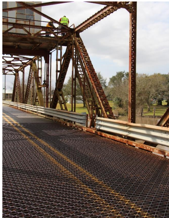
Condition Photo 15: Condition of metal grid deck on the swing span.
