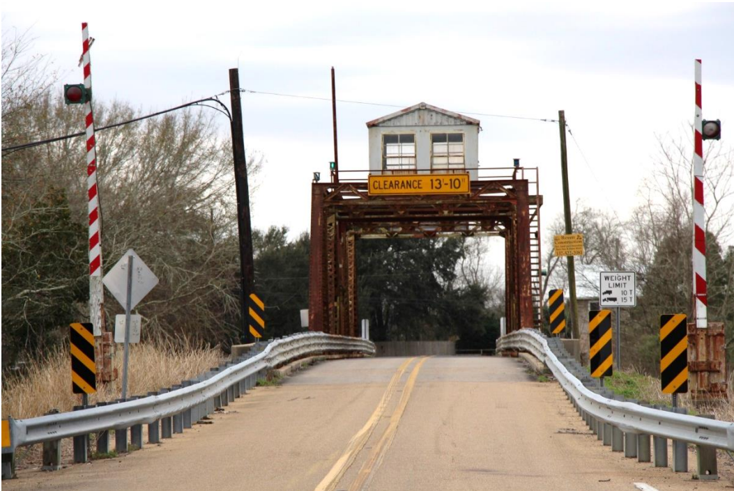
.Condition Photo 3: North roadway approach looking south toward the bridge. Note warning features and general view approaching the swing span.
