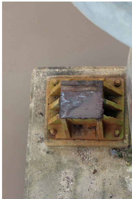
Condition Photo 11: Steel live load bearing for the main truss span.
